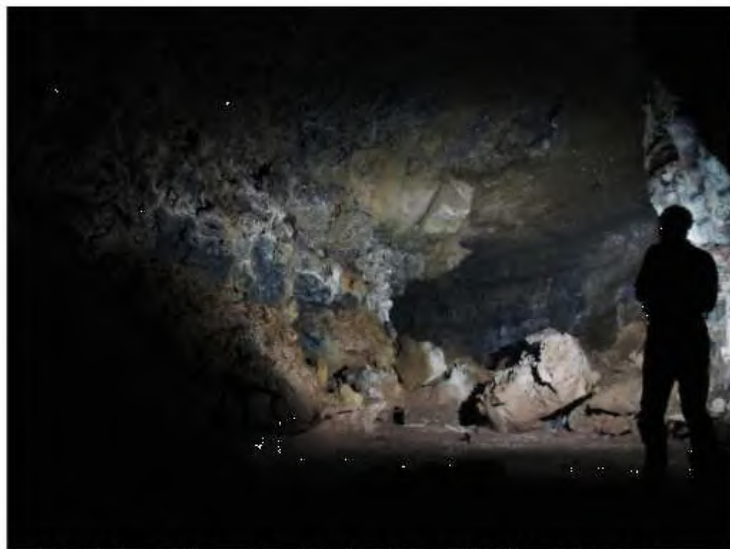
Fig. 15: View of the south wall below station Z2. To the right remains of the lining can be seen while to the left the eroded-into rocks are exposed, a series of pāhoehoe sheets covered by 'a'ā rubble (Photo: S. Kempe).
