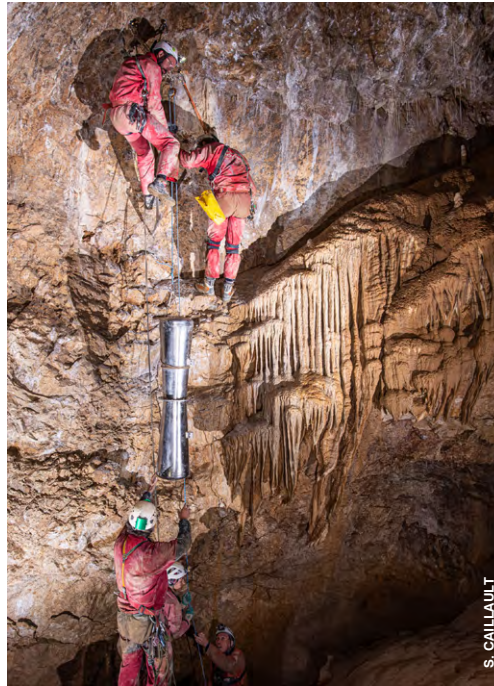
Installation of the time capsule on one of the walls of the Fitoja chamber. Climbing and installation was done without the use of metal anchors. The capsule and its anchor are made of stainless steel.
